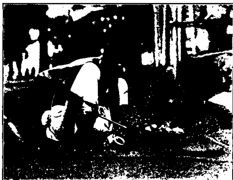
FIG. 2. BREAKING AWAY THE REMAINS OF THE SEPTUM FROM A SAWN CHANK CIRCLE (WORKING SECTION).
