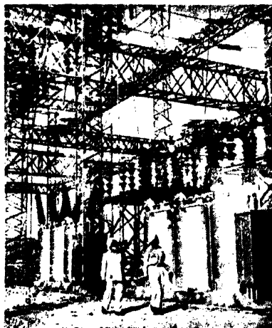
Power station at Bhakra-Nangal Project
