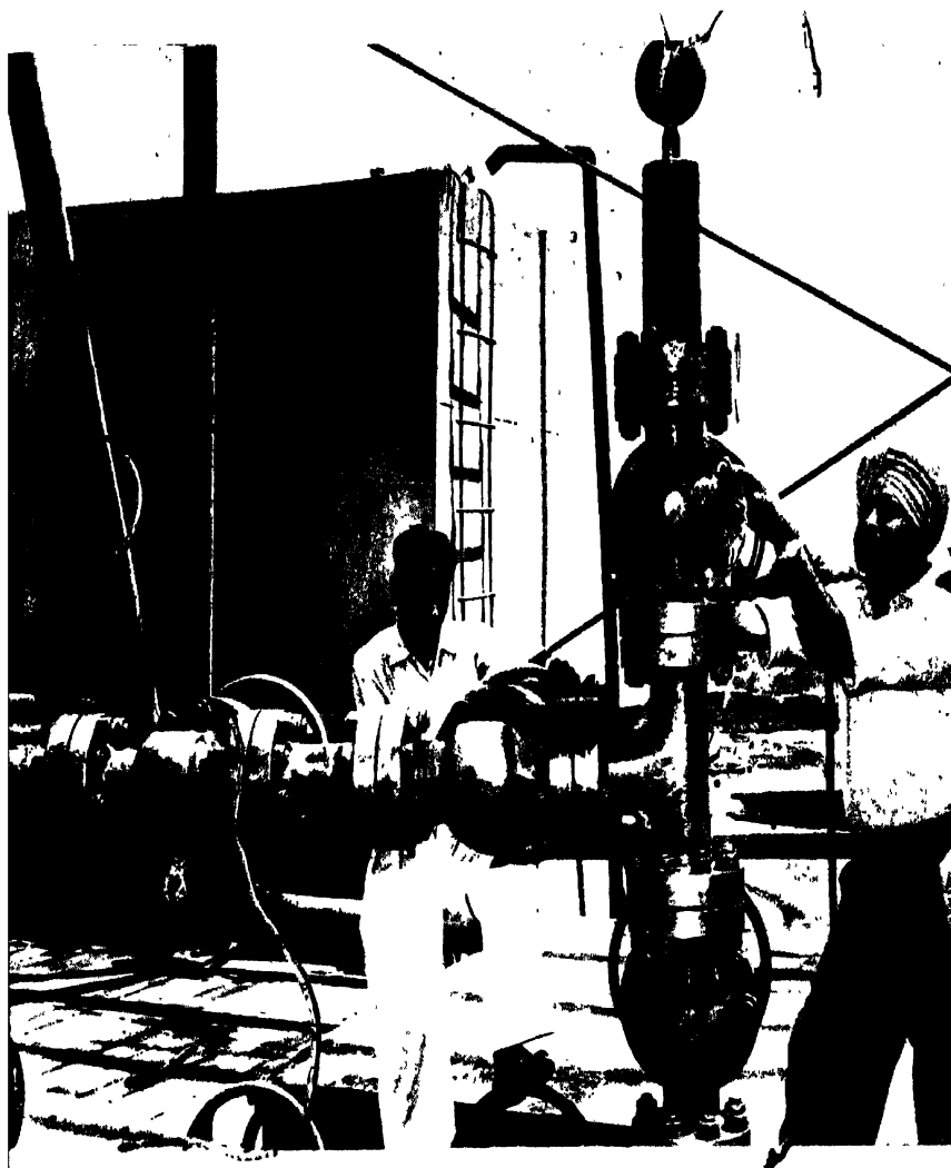
Large deposits of oil have been discovered in Assam and Gujarat. Three refineries are being established in the public sector. Technicians of the Oil and Natural Gas Commission are here adjusting the Christmas Tree valve at a test well at Kalol in Gujarat.
