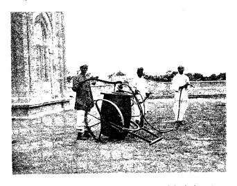
FIG. 48.—Barrel Pump. (Author's original photo.)
