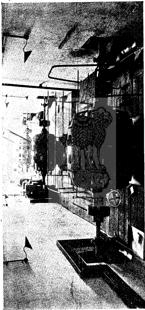
Electric Motors coupled to and driving the shafting in the Simplex Mill.
