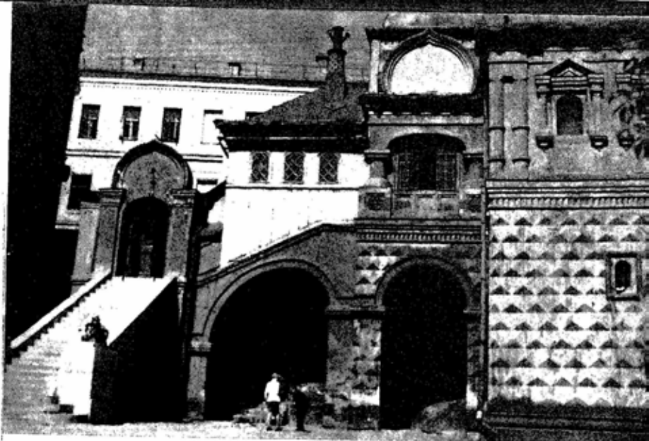
Plate 16, above A section of the Terem Palace built by the first tsars of the Romanov dynasty in the Kremlin at Moscow in the first half of the 17th century.
